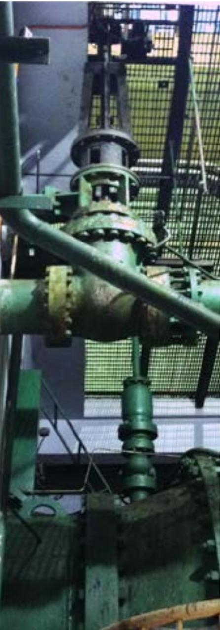
**PROBLEM:** If pressure is not balanced between both sides of the TIV, havoc can be wreaked on any unit. A turbine can experience turbulence, cavitation, and mechanical shock and fatigue that reduces the life of the equipment or disables it all together. The greater the pressure delta, the greater the risk. This makes the TIV Bypass a critical part of the startup sequence to equalize pressure.
