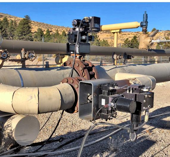
**KEY TO SUCCESS:** Maintaining injection well longevity requires monitoring and control of the fluid being injected back into the reservoir. Reliable flow control keeps fluid velocities high enough to prevent the settling of suspended solids and allows multiple units to feed a reduced number of injection wells. In flash plants, injection well flow control valves (often called Level Control Valves) are critical components that must accurately maintain back pressure and level in the separator.
