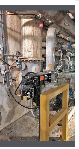
BACKGROUND: A REXA Electraulic™ Actuator was installed on a basis weight valve at a paper mill in the Northeast United States. An extensive benchmark test was performed to verify the REXA basis weight solution can meet or exceed the performance of the existing basis weight valve actuator. After eight months of run time, process data was collected to verify actuator performance.
