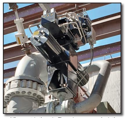
pneumatic actuation can increase ramp times, and if severe, trip the unit. The main governor valve is then opened wide for maximum load. REXA's **immediate response to signal change** and accurate control allows plant operators to reliably ramp up the vapor turbine, quickly connecting to the grid.
