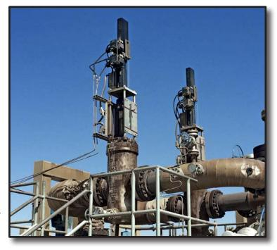
Reliable valve operation can also be a challenge due to silica and calcite scale buildup on internal parts. The ability to **power through** scaling with the force of hydraulics is extremely important to ensure the well head valves close when required. REXA Electraulic™ Actuation delivers the power and stability necessary to avoid unplanned shutdowns. Vibration, scale build-up and corrosion are no longer concerns for plant operators!
