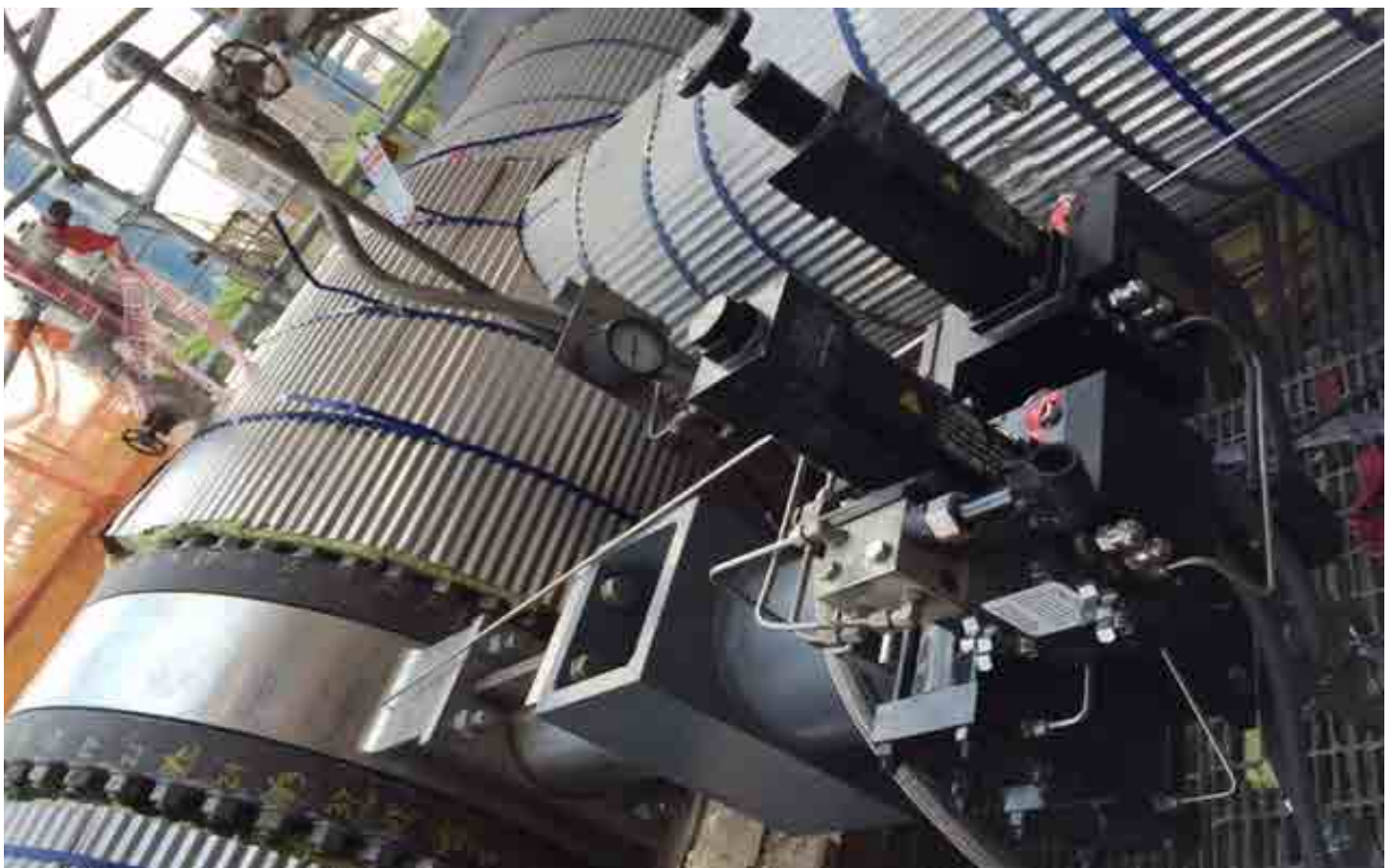
Fully Redundant REXA Actuator on Flue Gas Butterfly Valve
