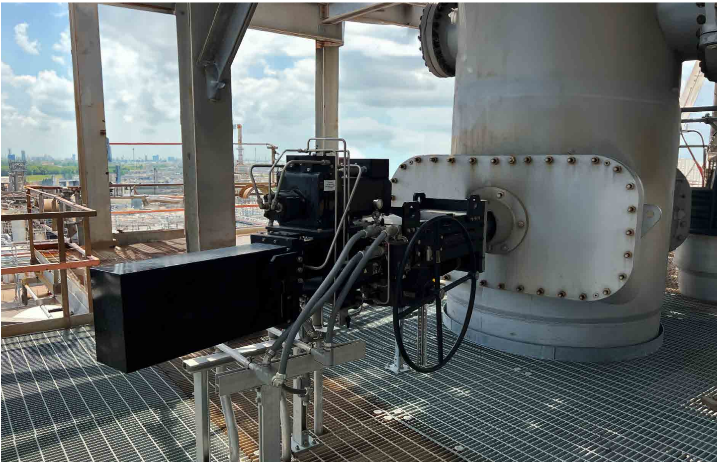
REXA Actuator on Flue Gas Double Disc Slide Valve
