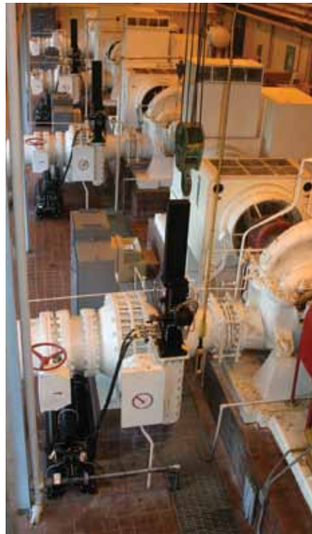
The self-contained actuators incorporate hydraulic, electronic and mechanical technologies. There are two main components – the Electraulic power module and a control enclosure.
