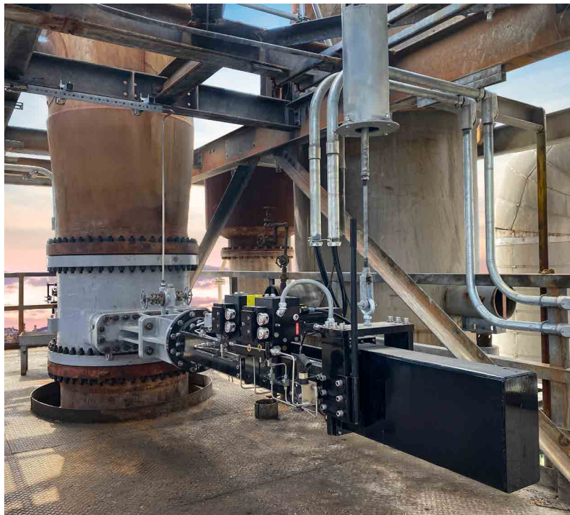
Linear Double Disk Slide Valve
