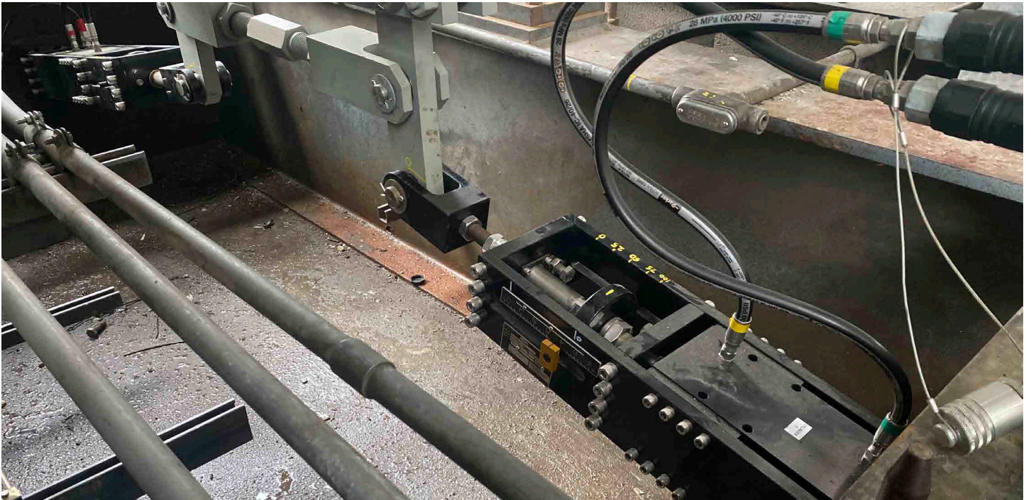
Compressor Inlet Guide Vane Control
