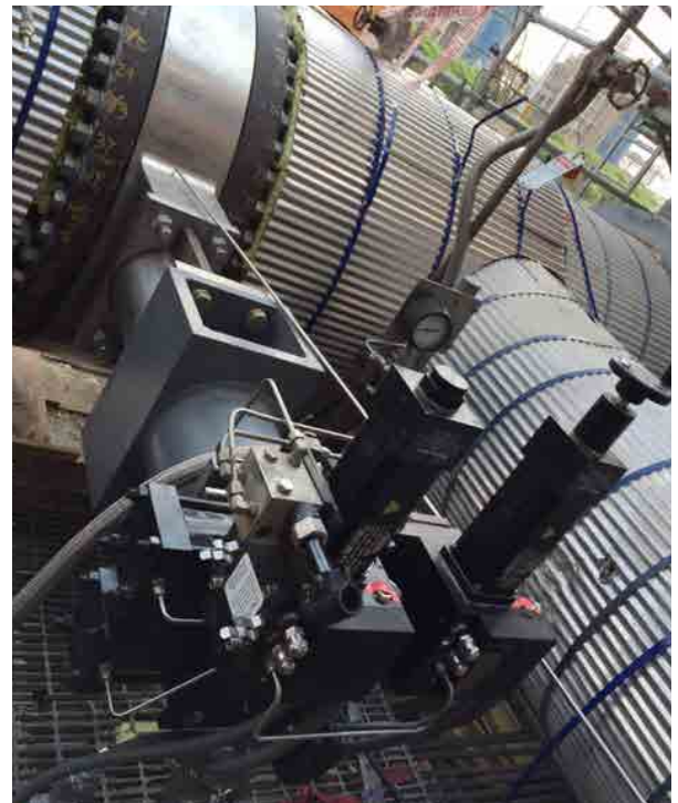
Rotary Butterfly Valve(s) (recycle to expander)
