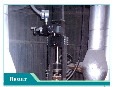
Upgrading from pneumatic actuators to REXA Electraulic<sup>™</sup> Actuators on feedwater control can garner immediate benefits for any power plant. Maintenance savings can be immediately realized through improved trim life of the control valve, reducing labor and material costs.
