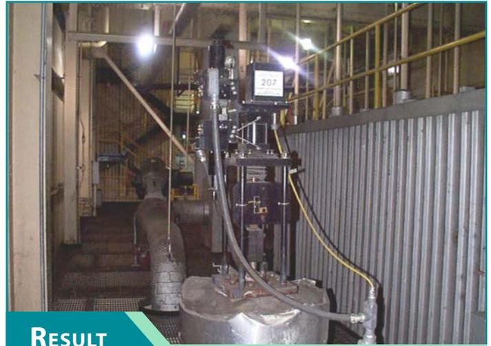
A supercritical plant operator will immediately notice smooth ramping startup valves that don't jump, stick, or overshoot. Putting a startup valve into auto mode for the first time is not uncommon. The ability to throttle bypass and level control valves at minimum travel becomes normal, thanks to 70mS deadtime, and a resolution of <0.1%.
